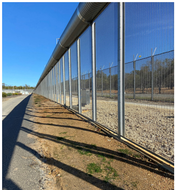
Figure 3: YHIDC perimeter fences
